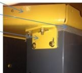
Foam Gasket A/C Mount Bracket And Bolts (both sides)
