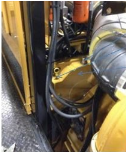
Vented Fill Plug Pump Drive Dipstick Pump Drive
